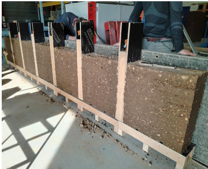
Rammed earth samples built for future tests
