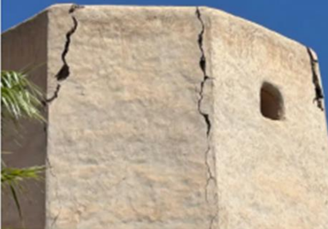
Earth building in Marrakech with restoration intervention after the earthquake (photograph: Montserrat Villaverde)
