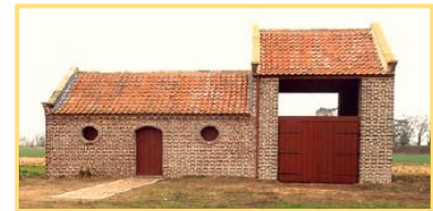
Stephen Pickering, 2016 (18 th century) Repaired with hot mixed air lime mortars
